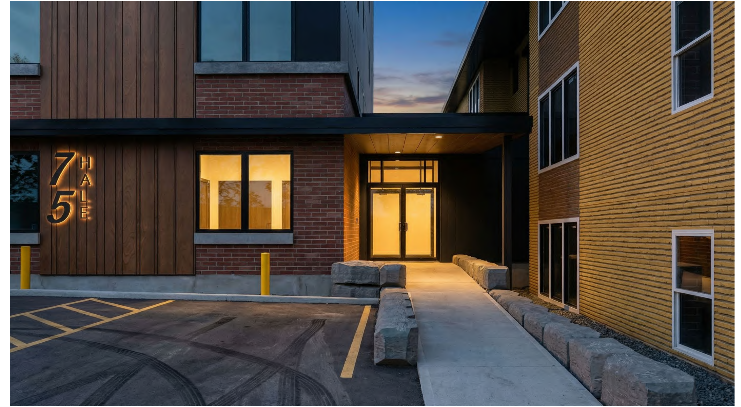
A sloped sidewalk leads to the main entry located in the breezeway connecting the new and existing building.
